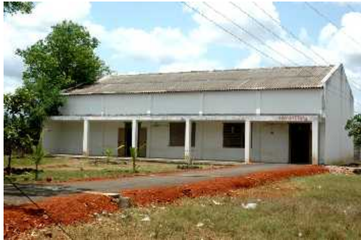
EEE Laboratories Block
